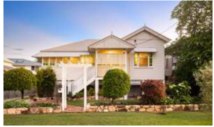
24 Junction Street, Sherwood
